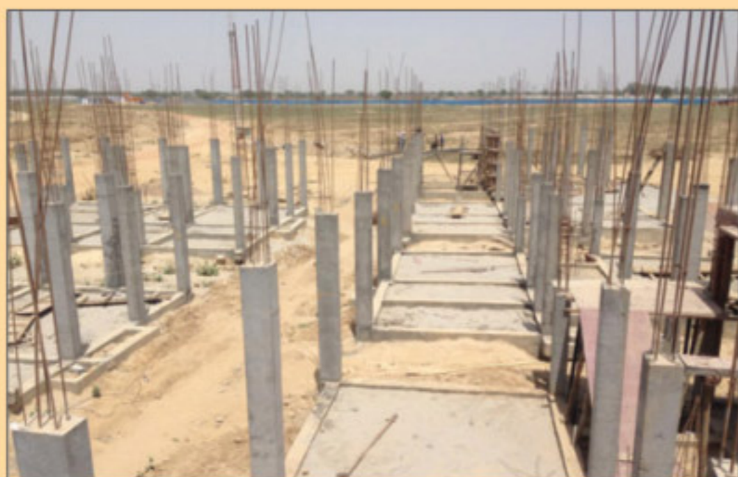
Column RCC completed in B and C type villas
