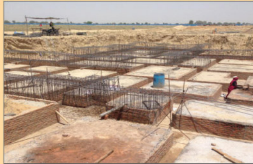
D type (3 BHK) foundation beam reinforcement placing in progress
