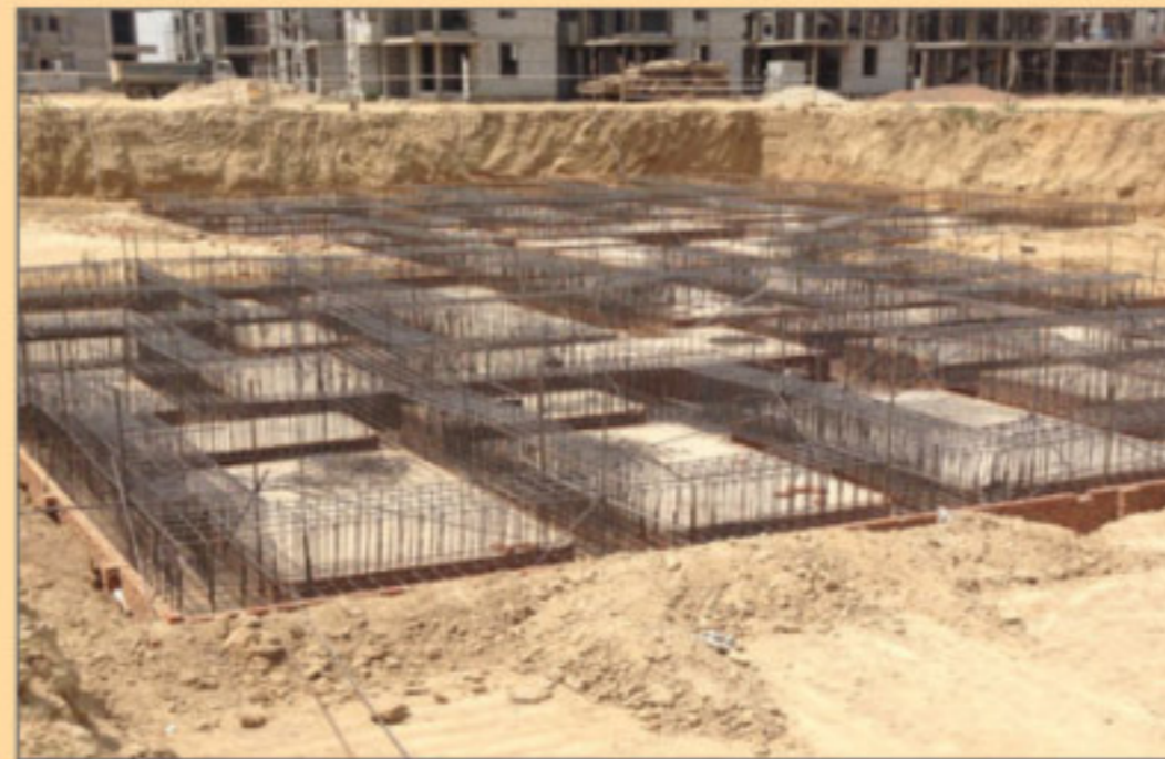
G type tower (studio) foundation beam reinforcement work in progress
