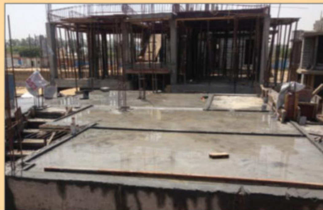
C5 1st floor slab RCC completed
