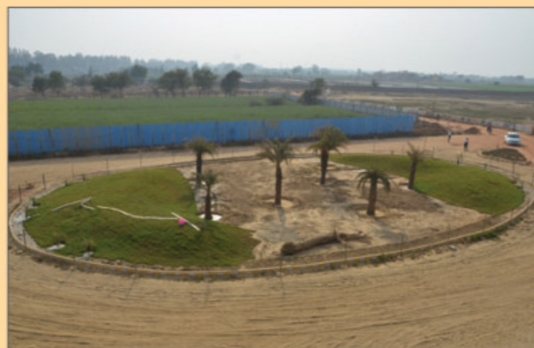
Residential entry of Krishna bhumi work in progress
