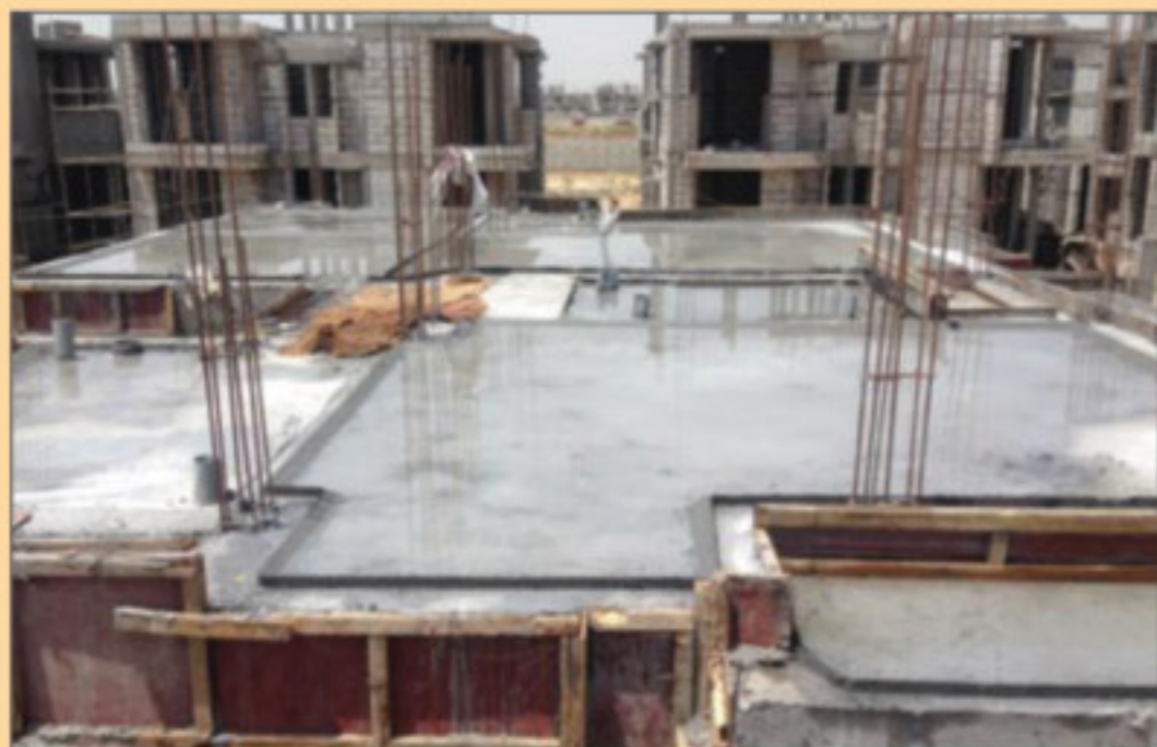
B9 1st floor slab RCC completed
